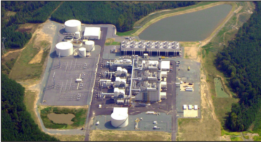
The 885 MW Tenaska Virginia Generating Station near Scottsville, Va., is a natural-gas fueled plant that produces electricity in an environmentally responsible manner.
